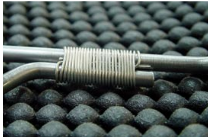
A good mechanical joint is created by tightly wrapping the joint with fine copper wire. Try to keep the wrapping neat and tuck the ends under the wraps.
